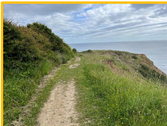
Eroding cliff top creating pinch point in coastal path. (/0201C01)
