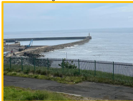
No Access - Tipped rubble (/0104C16) and rock revetment (/0104C01)
