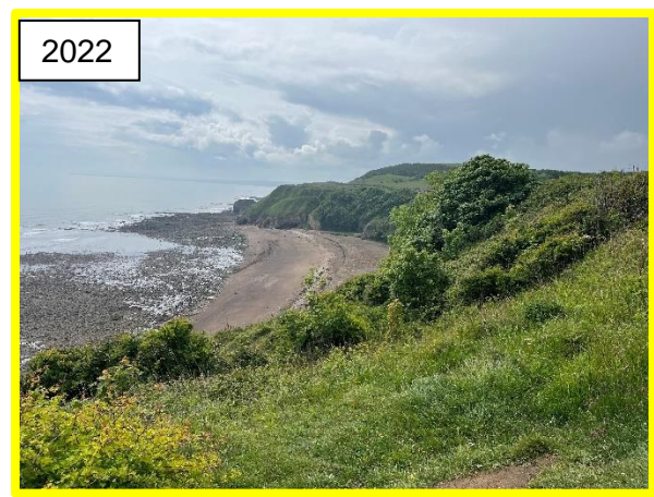
Residual spoil beach at Hawthorne Hive – 2022 (/0201C01)
