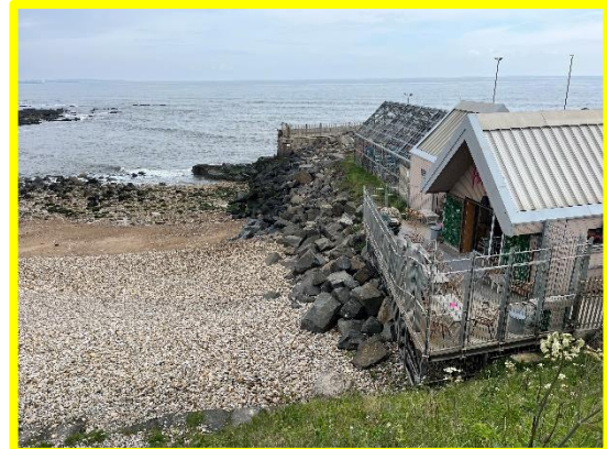
Revetment preventing outflanking of the North Pier(/0104C02)
