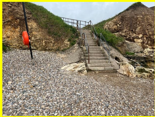
Access steps adjacent stone revetment (/0804C01)
