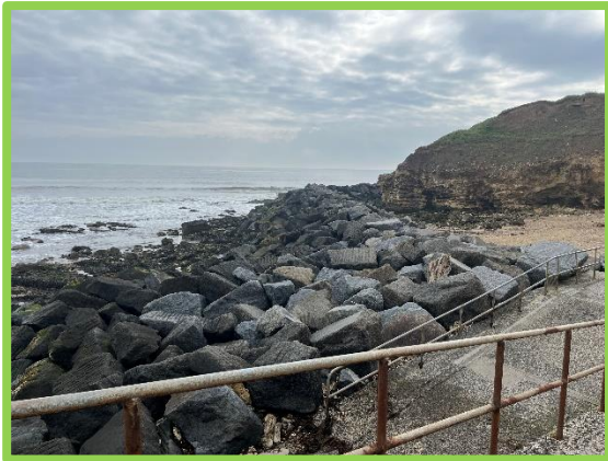
Rock berm around Featherbed Rocks headland (/0103C01)
