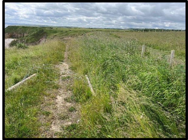
Previous cliff failure through coastal footpath. Fence to prevent access has failed (/0201C01)
