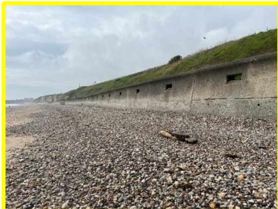
Northern section of Seaham sea wall with minimal abrasion (/0102C01)
