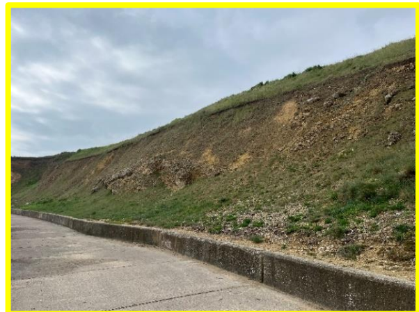
Headscarp in backing cliffs formed by previous slippages (/0102C01)
