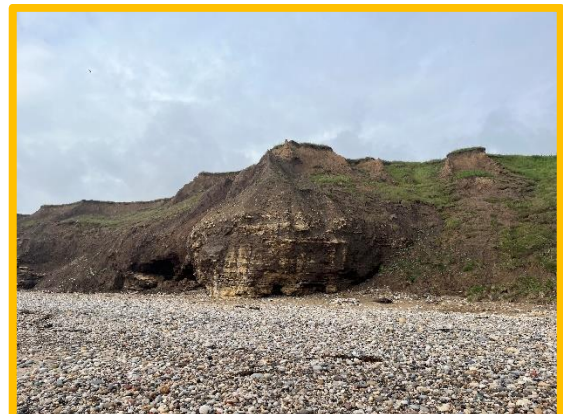
Localised slumping of upper till within the cliffs (/0804C01)
