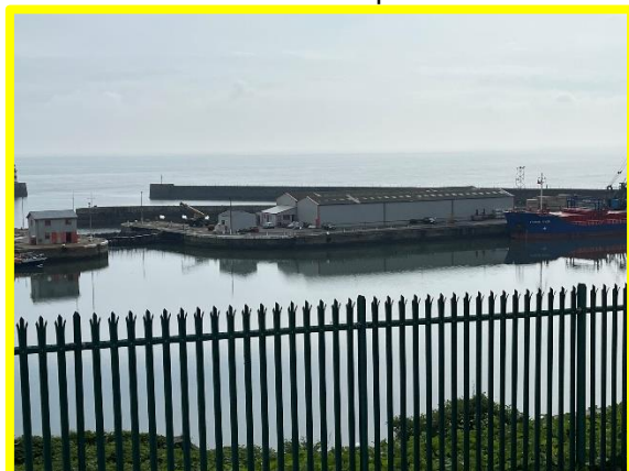
No Access - Seaham Harbour South Pier (/0104C17)
