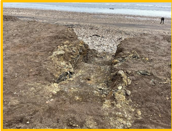
Informal access steps benched through the colliery spoil (/0201C02)
