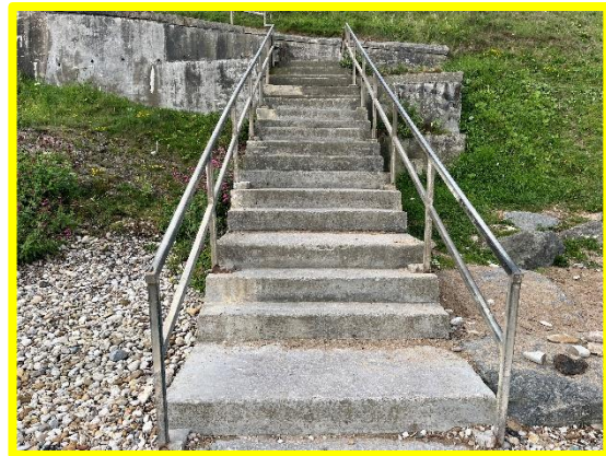
Access ramp and steps (/0103C07)
