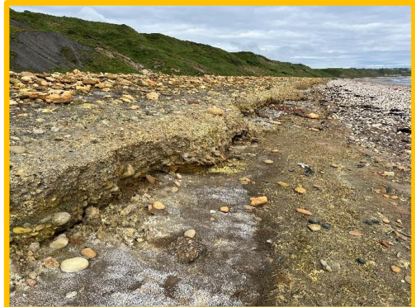
Minor erosion to colliery spoil to the south of the bay (/0201C02)
