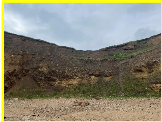
Small scale failures to North face of Featherbed Rocks headlands (/0103C01)
