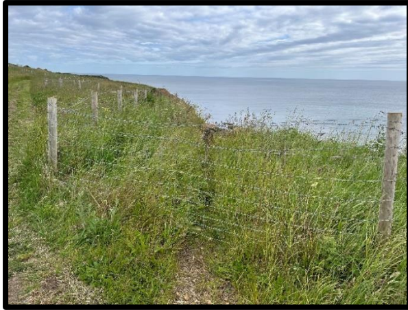
Previous cliff failure through coastal footpath fenced off (/0201C01)
