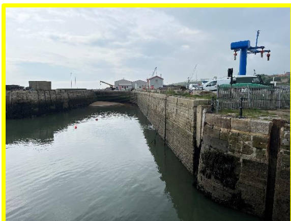
Inner face appeared in good to fair condition (/0104C10)
