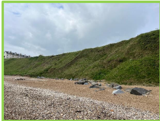
Local slumps in cliffs (/0103C06)
