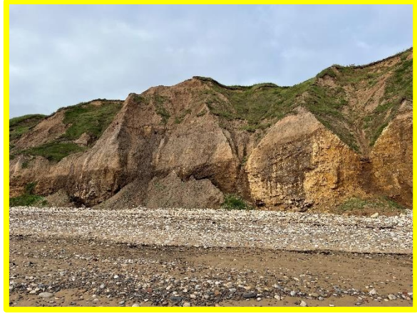
Large-scale slump of softer material (/0301C01)
