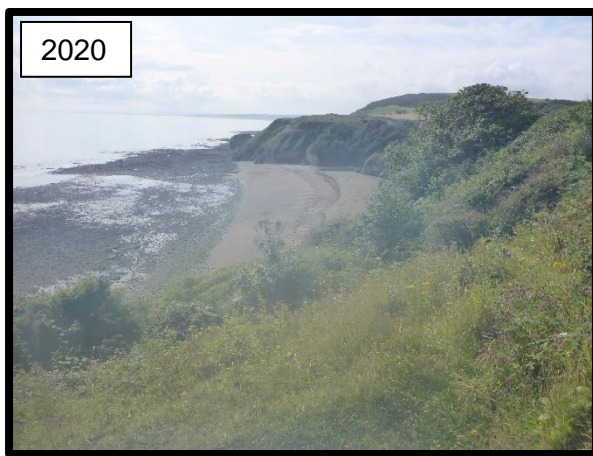
Residual spoil beach at Hawthorne Hive – 2020 (/0201C01)
