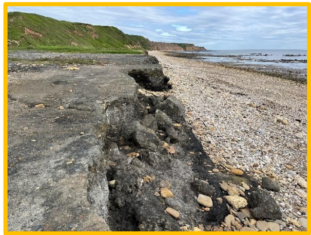
Significant ongoing erosion to the colliery spoil to the North of the bay. Note – tension cracks and debris piles (/0201C02)
