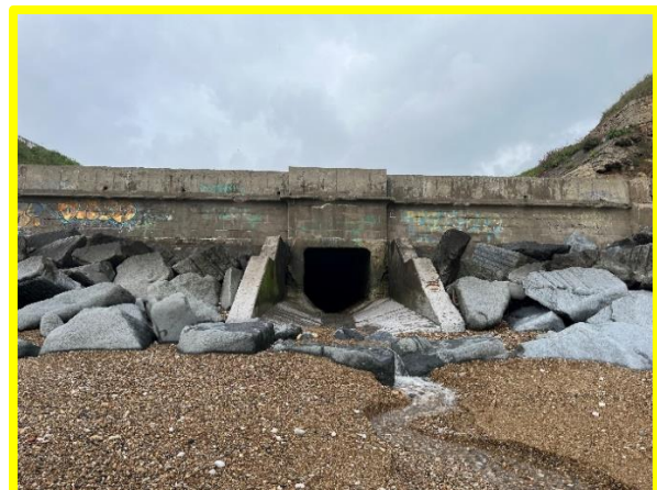
Rock berm around Dawdon Dene culvert and further south (/0103C04)
